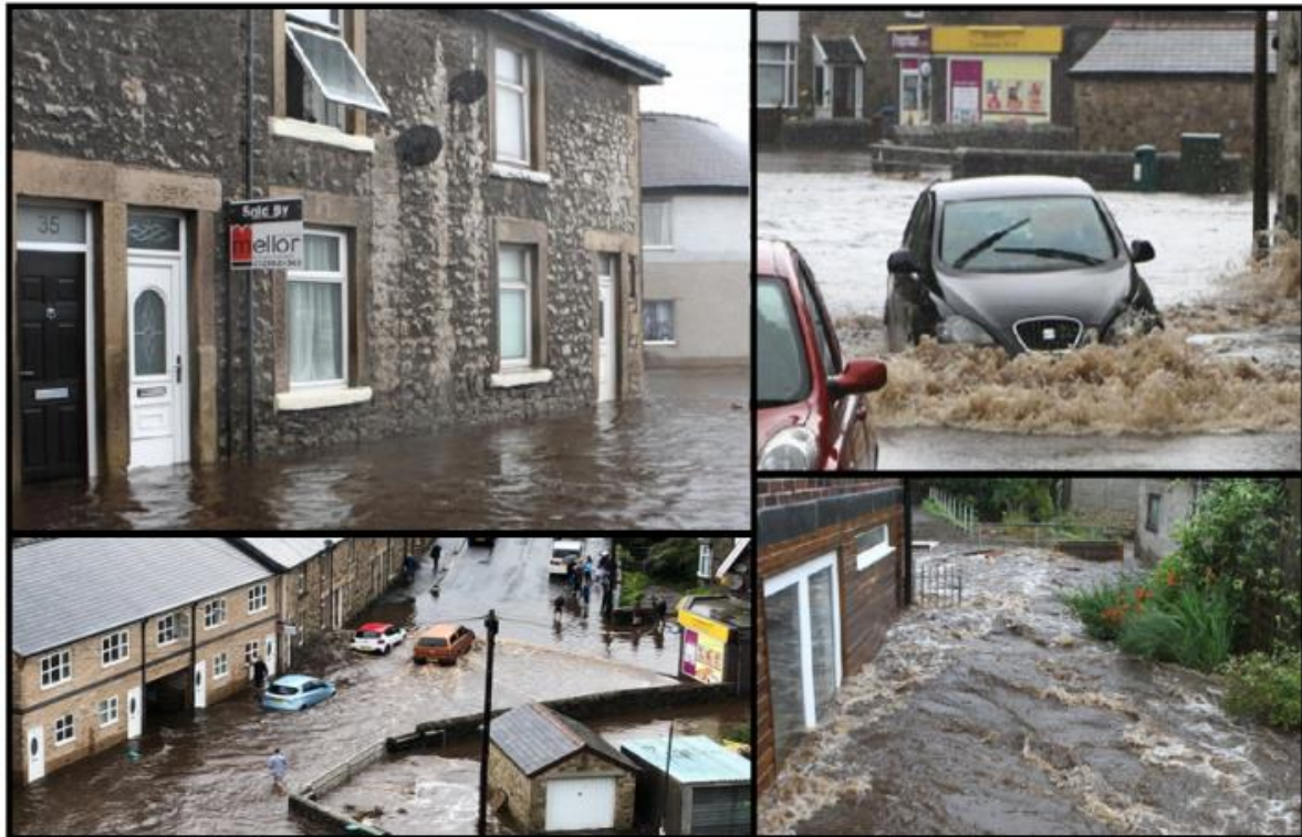
Figure 7: Photographs taken of the flooding (Lightwood Road) on 31st July 2019
